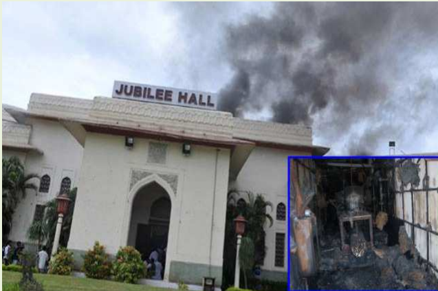
Fire incident at Jubilee Hall (Inset: burnt AC plant)
