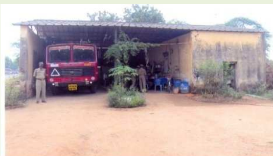
Gadwal-FS building in a dilapidated state (10 November 2011)
